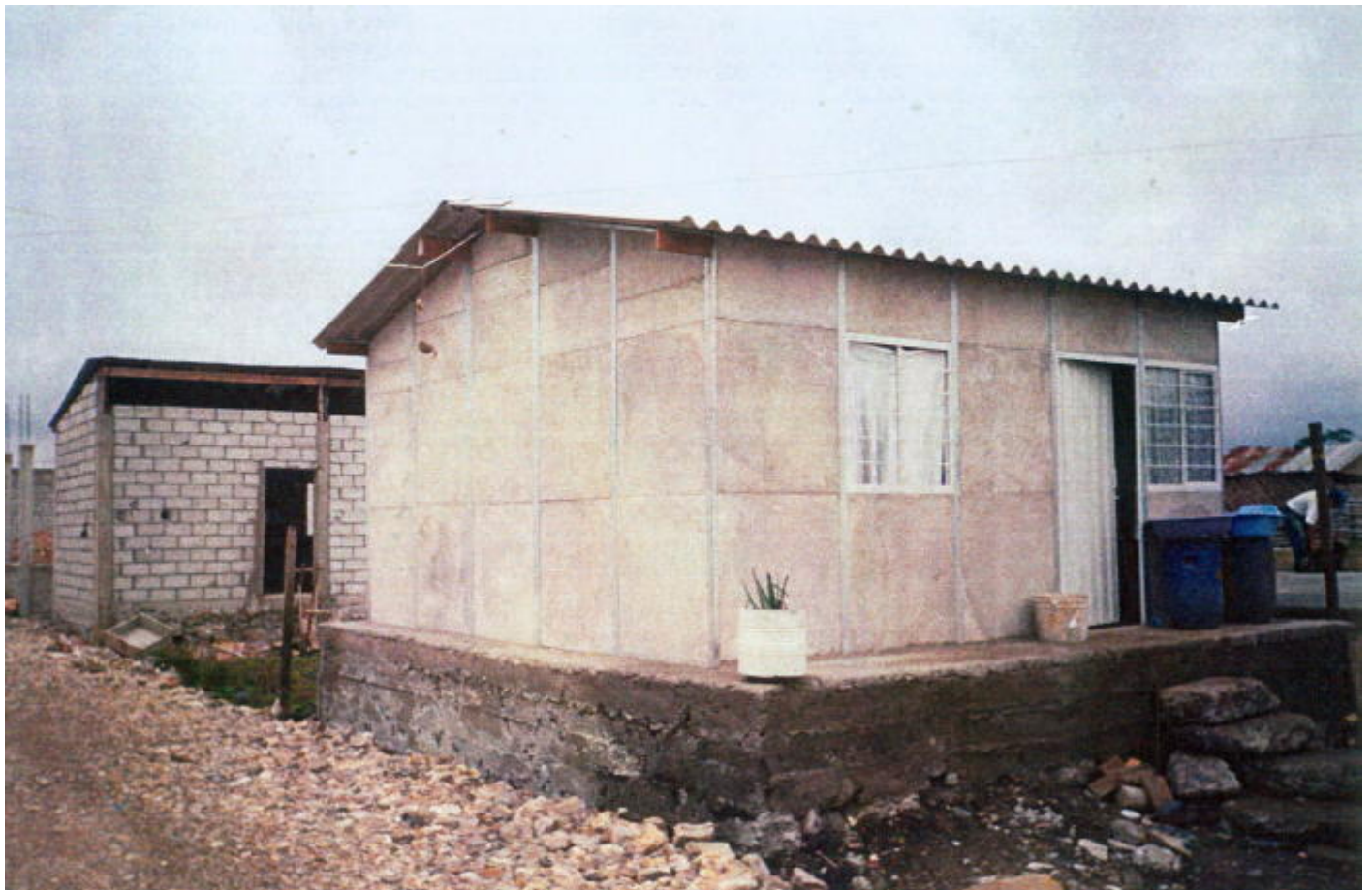
Step 5. Use pre-fabricated panels to build walls. Different sizes of panels are required near door and window openings. Conventional roof methods were used to complete the building.
