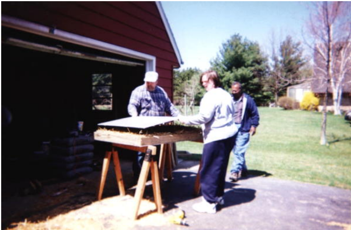
Step 5. Use pre-fabricated panels to build walls. Different sizes of panels are required near door and window openings. Conventional roof methods were used to complete the building.
